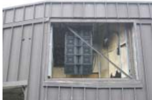
Pro Sound Service installed new JBL VERTEC line arrays in the Tweeter Center in Mansfield, MA.
