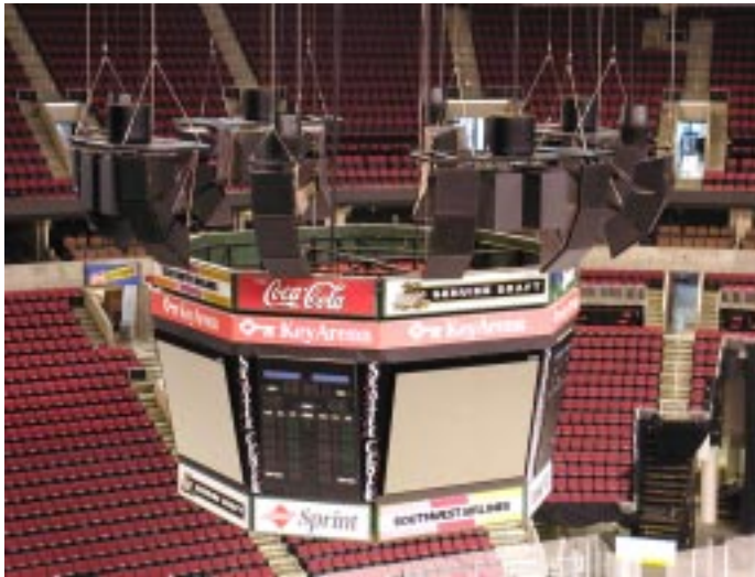
Eight PD Series Arrays Form a Ring Around the Scoreboard at Key Arena, Seattle, Washington.
