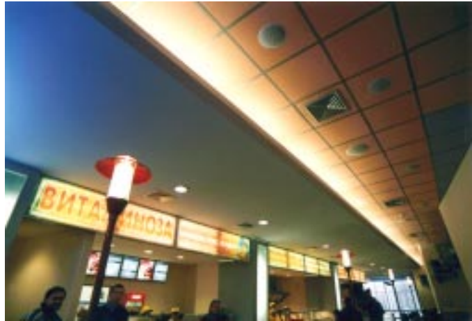
Control Contractor speakers installed throughout the facility, including the lobby (above) and the childcare center (below).
