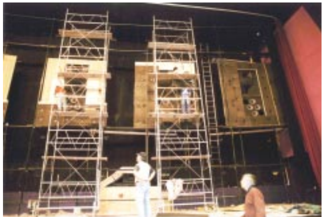
JBL 5674 three-way speakers during installation.
